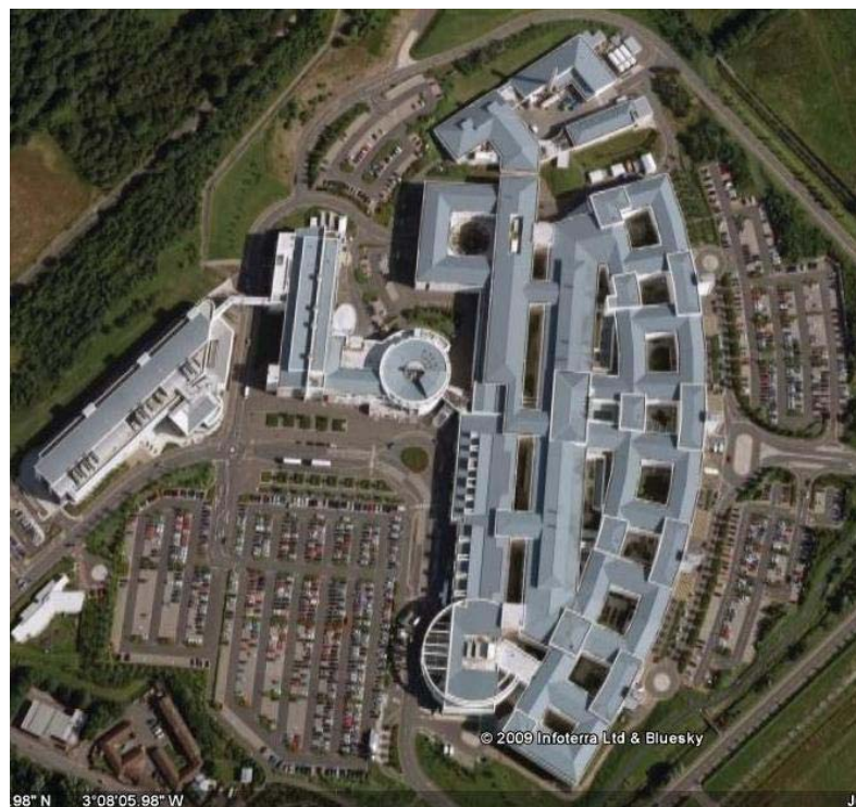
Figure 7 Aerial view of the new Royal Infirmary Edinburgh. Building provided by Consort healthcare and Balfour Beatty workplace.
